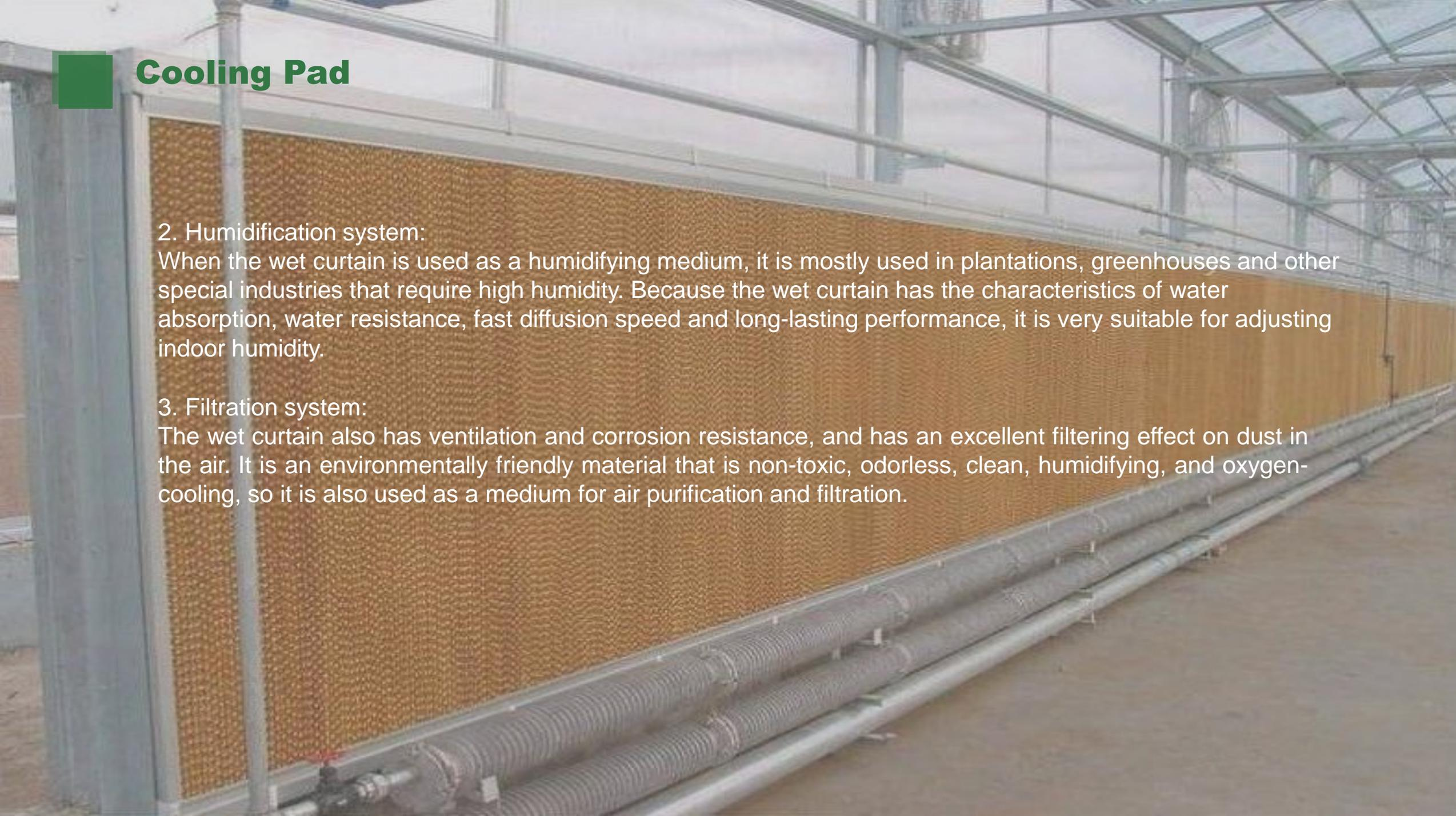
A photograph showing the interior of a greenhouse. The structure is made of a metal frame with a translucent plastic covering. A large section of the wall is covered with brown, textured cooling pads. Below the pads, several grey, corrugated pipes are visible, likely part of a water distribution system. The floor is a light-colored concrete or dirt.
